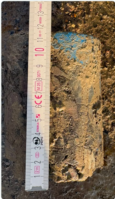
The core from chainage 150, centre line.
